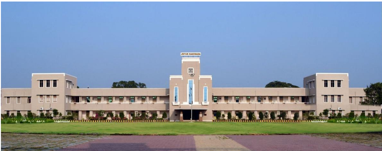
Figure 1 Administrative building of JNTUK Kakinada
